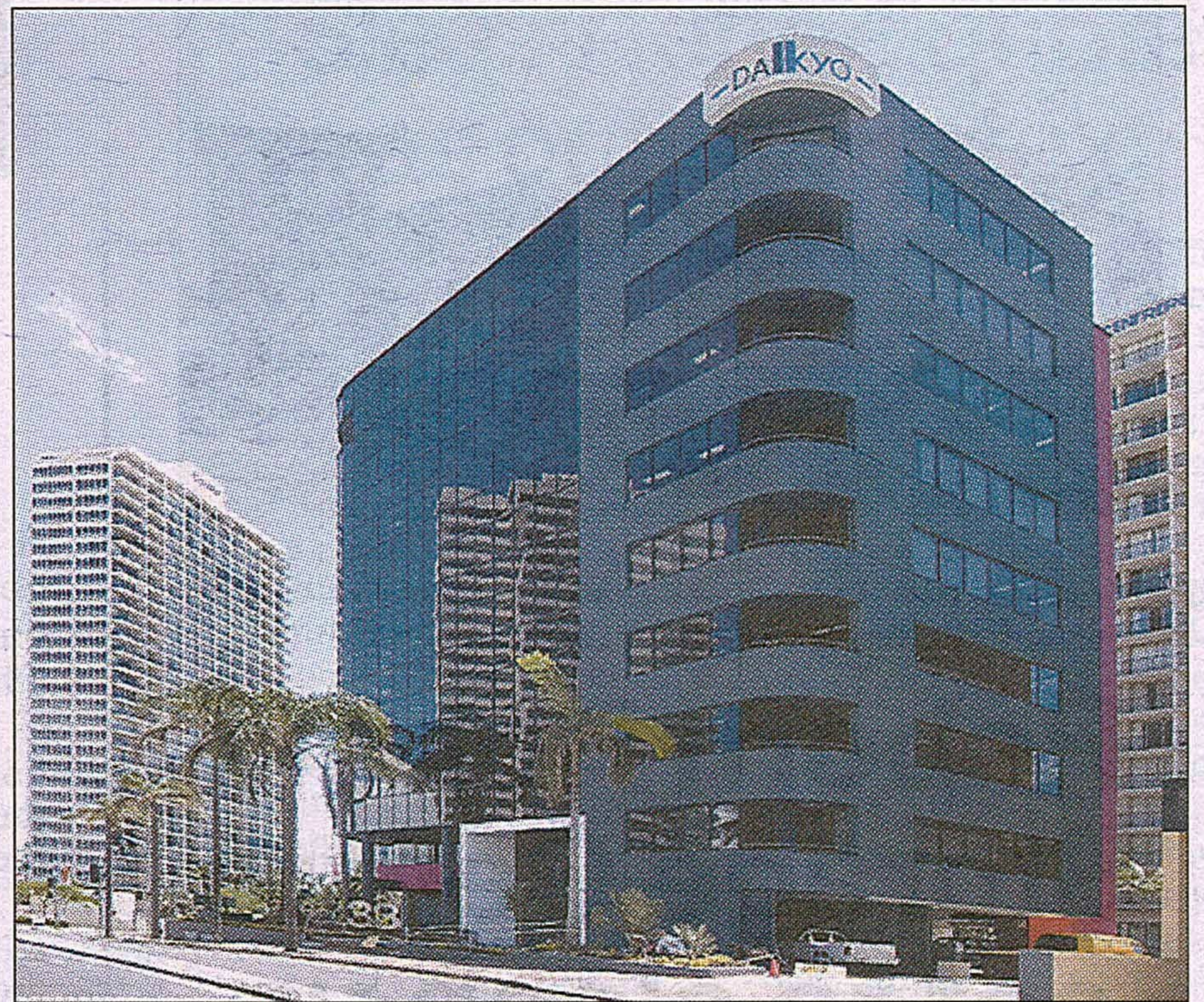
Above: 33 Elkhorn Avenue . . . soon to be home to Bayliss and Samra Commercial Realtors
